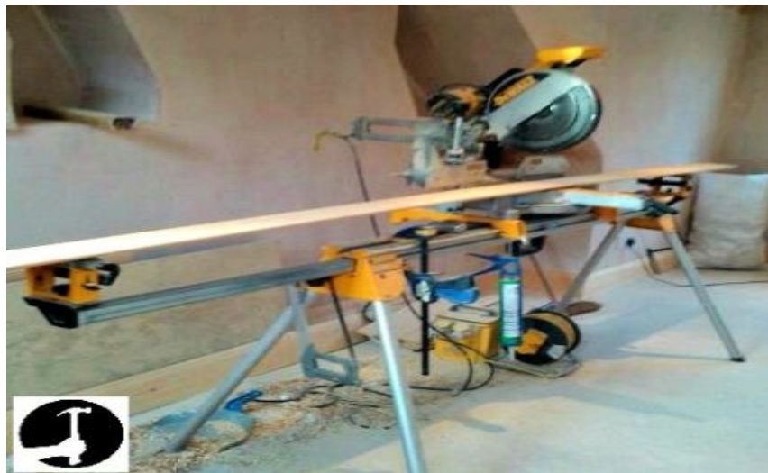
Figure 8 fitting skirting materials
